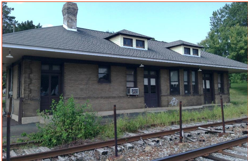
SELLERSVILLE TRAIN STATION
