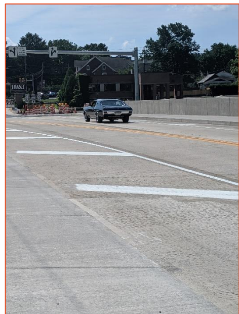
MAIN STREET BRIDGE
