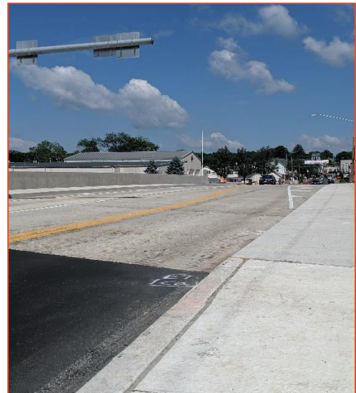
NEW MAIN STREET BRIDGE
